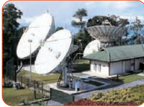
MEASAT's Satellite Control Centre
