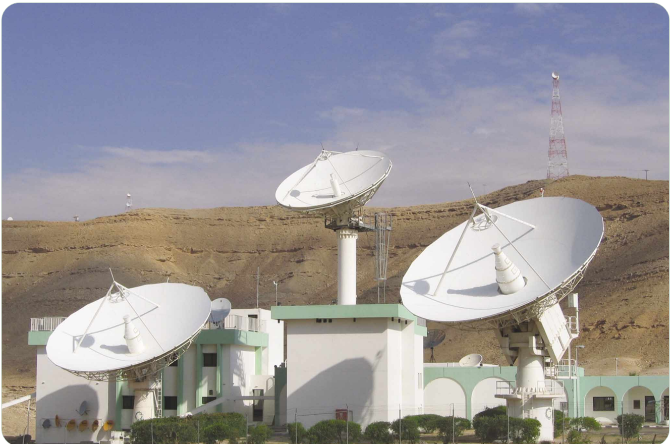
ArabSat Riyadh earth station.
