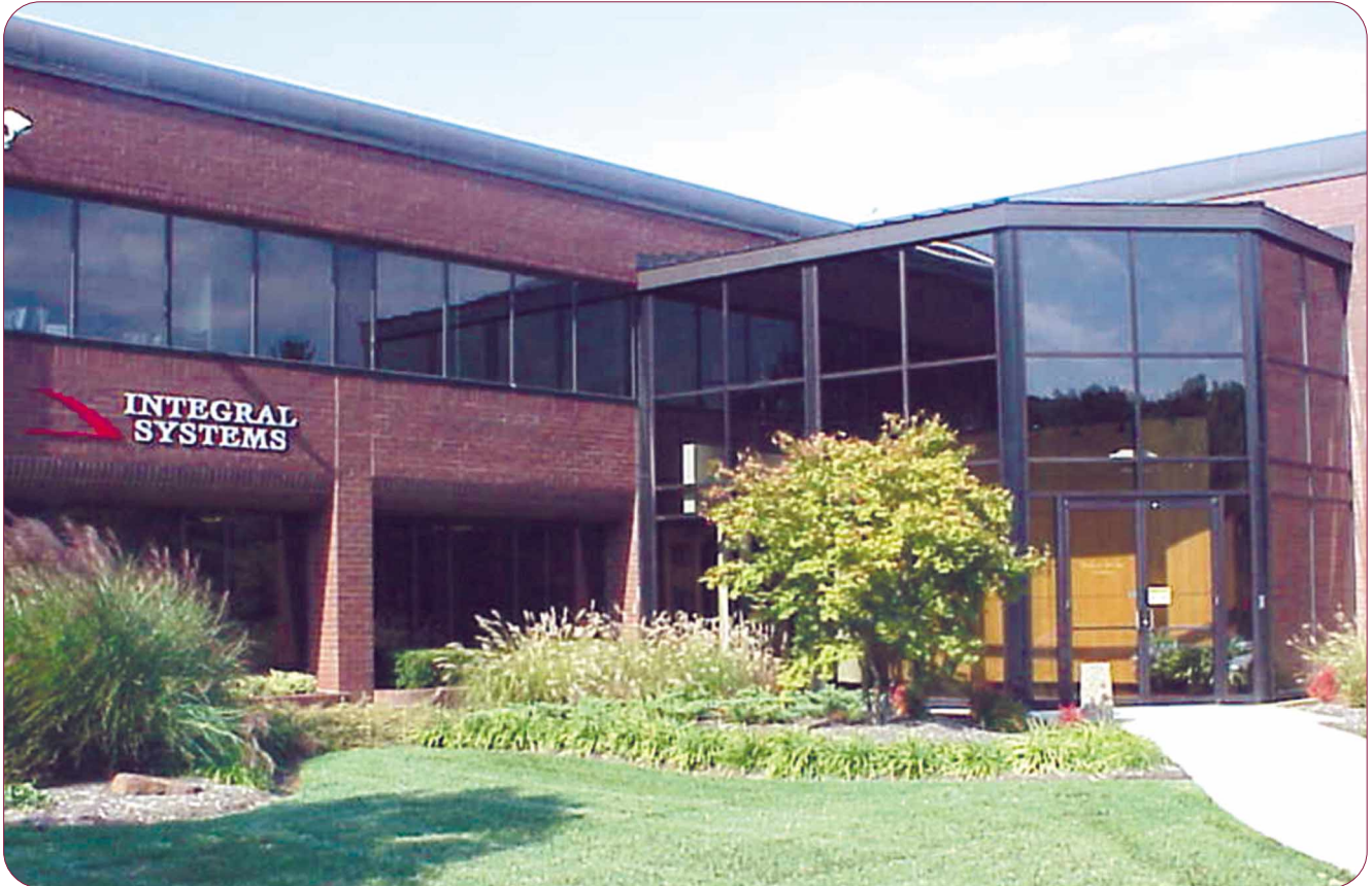
Integral Systems HQ. Photo courtesy of Integral Systems
