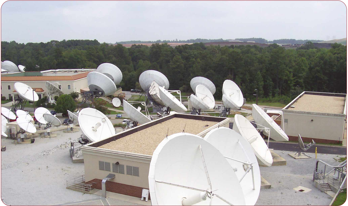
Teleport in Ellenwood, Georgia. Photo courtesy of Intelsat.
