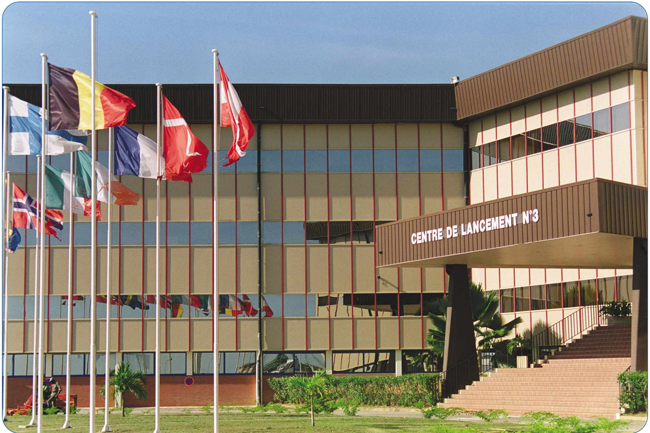
ELA-3 launch control room for Ariane 5 (exterior view). Photo courtesy of Arianespace.
