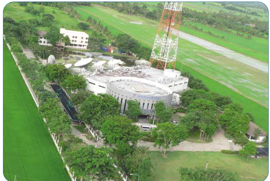
THAICOM teleport and DTH centre.
